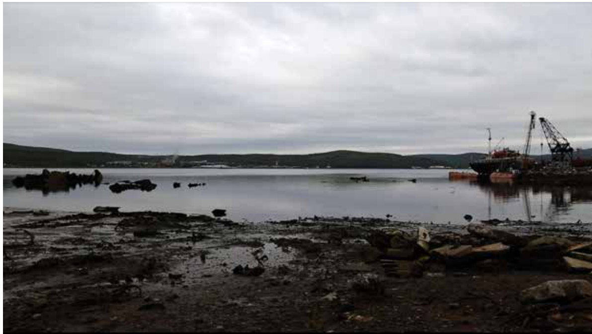
The All Infrared Line , film still, 2014. Potential Russian ROTACS cable landing point in Murmansk harbour.
